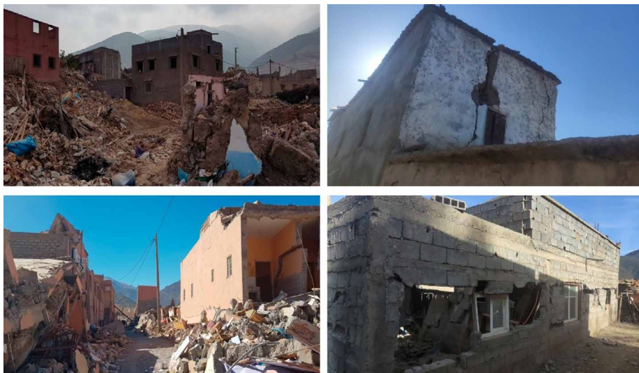
Figure 4 Impact of Masonry Quality and Structural Detailing on the Seismic Response of Stone Masonry Buildings: Insights from the Al Haouz Earthquake.
