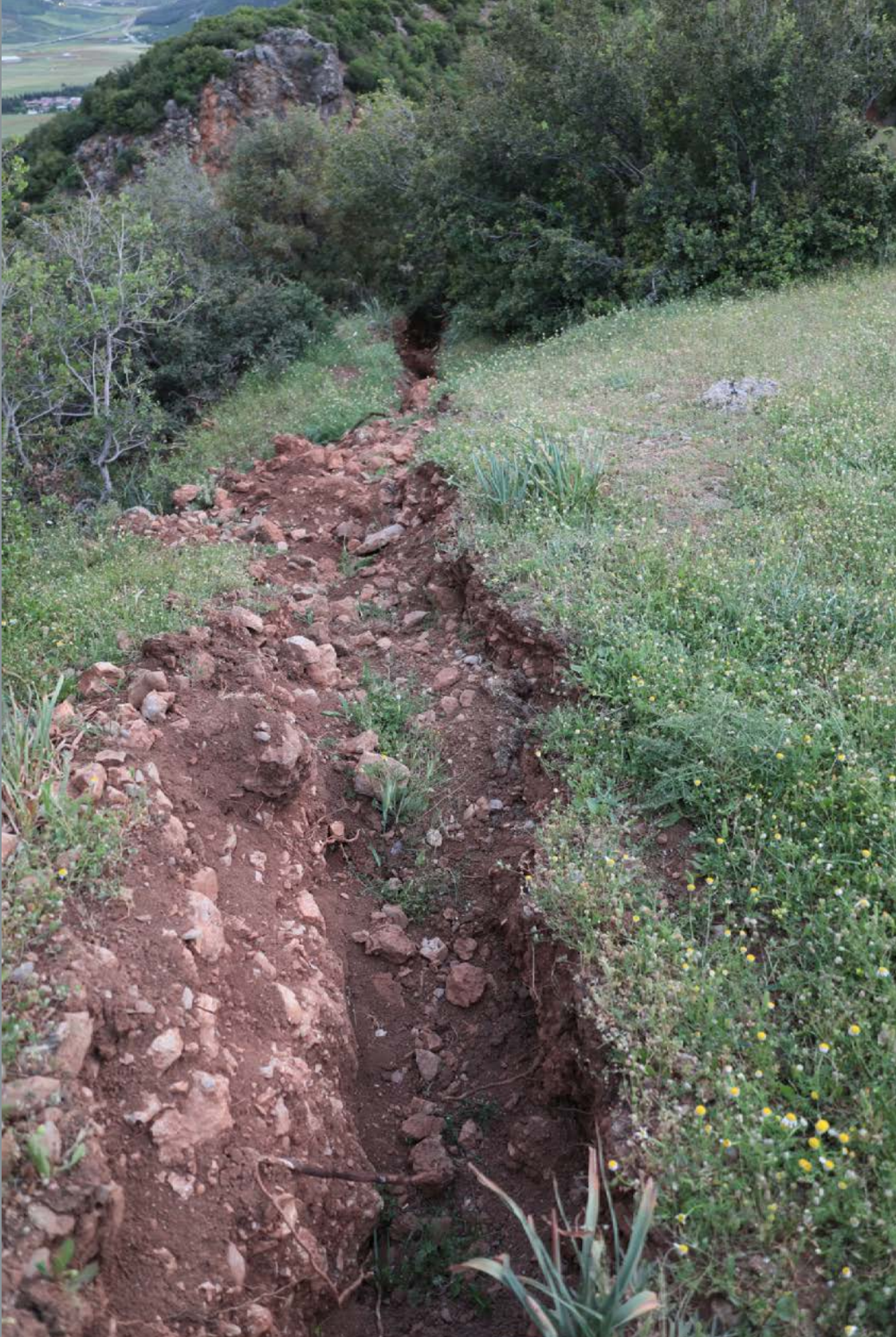
Photo 6 (37.140567°N, 36.681057°E) – The mole-track pattern is characterised by transtensional fractures with up to 60 cm of opening component, resulting in a trench up to 2 meters deep, frequently infilled by gravitational collapse of the two walls.
