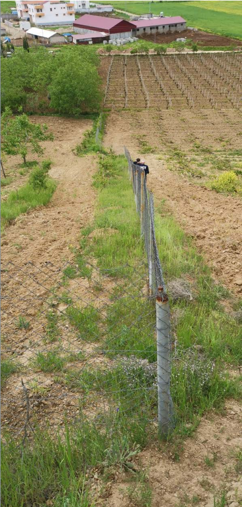
Photo 86 (37.728819°N, 37.554887°E) – Fence dislocated by the left-lateral strike-slip fault (view from northwest).
